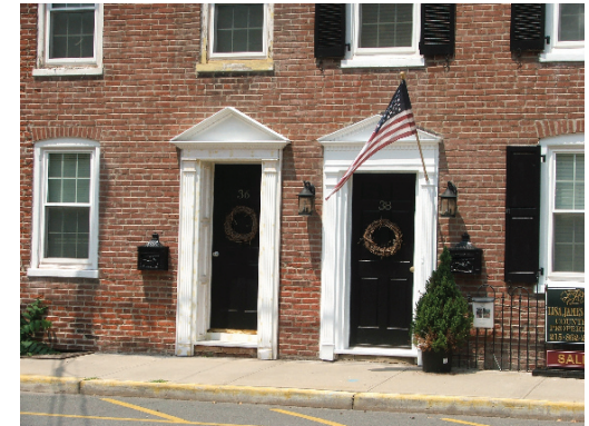
The door on the left was recently constructed on this house when the house changed from a single family structure back to a duplex. Although the details are very similar to the original 19th century door on the right, the subtle differences are important for understanding the difference in time periods.
