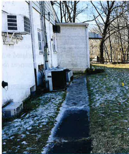
6 - Asphalt pathway on north side of the building
