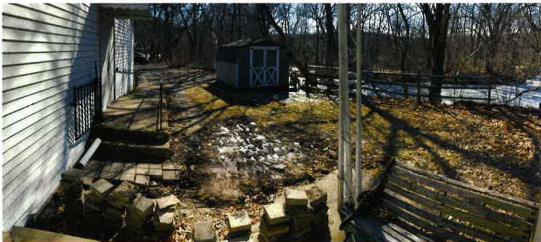
7 - Remnants of the paver walkway at rear of the building
